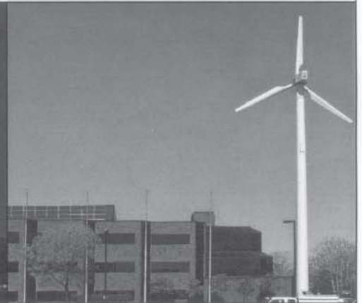
JATC Training Center/Wind Turbine, Boston, MA
