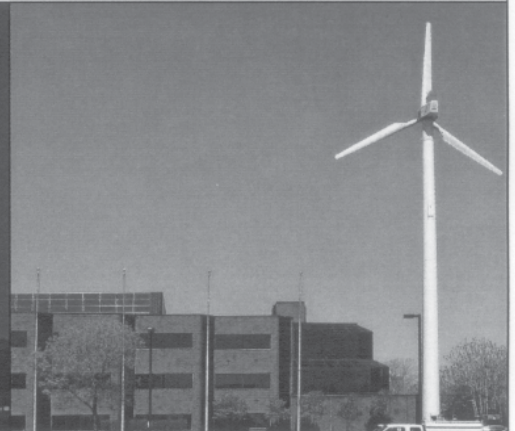
JATC Training Center/Wind Turbine, Boston, MA
