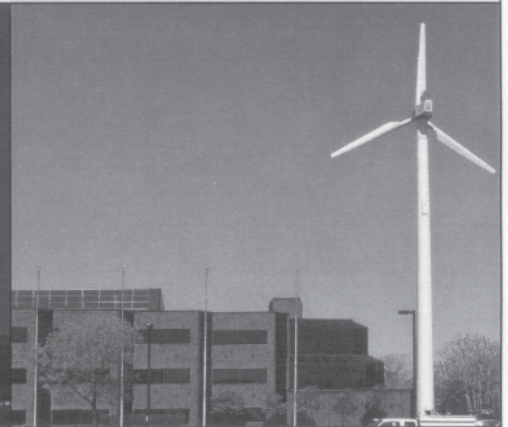
JATC Training Center/Wind Turbine, Boston, MA
