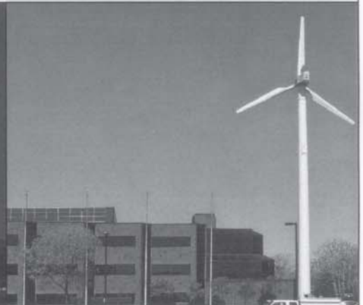
JATC Training Center/Wind Turbine, Boston, MA
