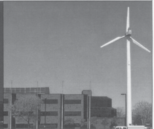
JATC Training Center/Wind Turbine, Boston, MA
