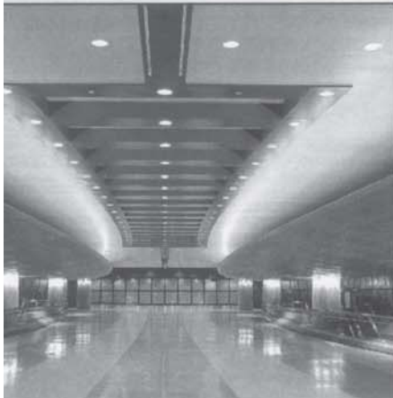
House Station, Silver Line, Boston, MA
