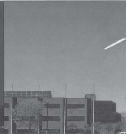
JATC Training Center/Wind Turbine, Boston, MA
