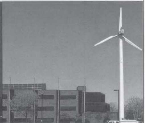
JATC Training Center/Wind Turbine, Boston, MA
