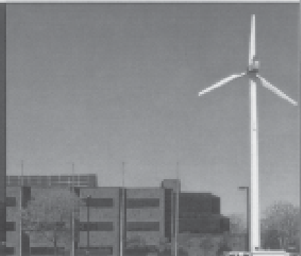
JARC Training Center/Wind Turbine, Boston, MA
